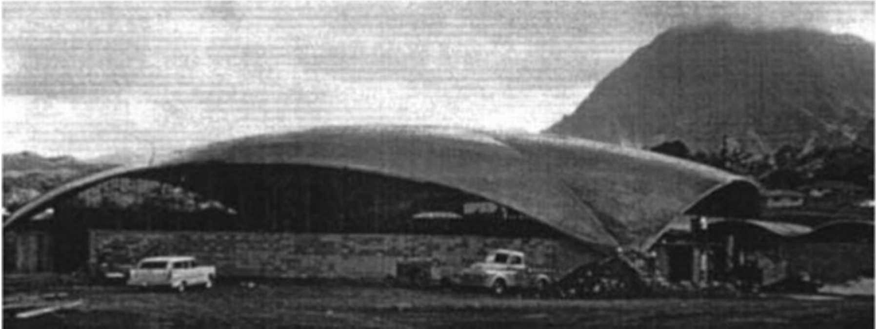
Torus Shell – R. Bradshaw – 37m span – 64 to 127mm thickness without ribs
