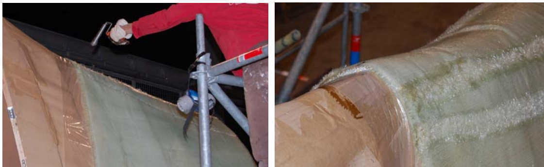
Fig.11 – The cut was repaired with a single layer glass mat
