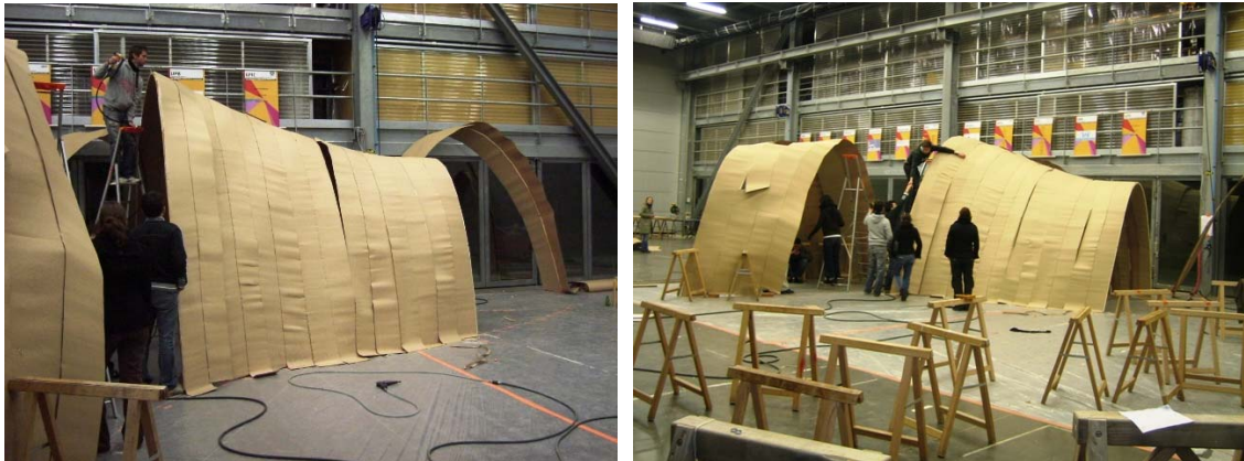
Fig.7 – General assembly of the cardboard free form
