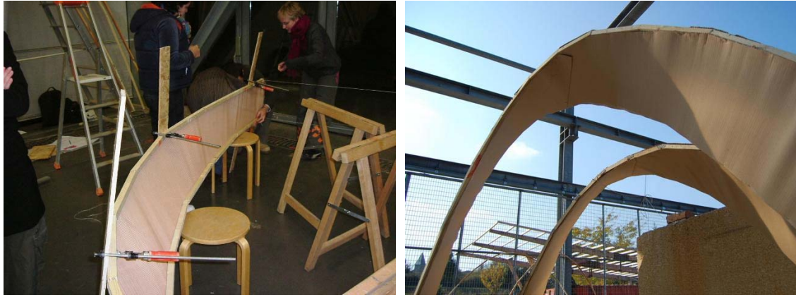
Fig.6 – Assembly of wooden parabolas and cardboard panels
