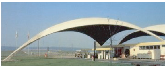
Figure 8-a. Gazoline station, Deitingen, Switzerland, 1968.
