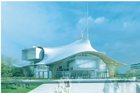
Figure 15-a. Centre Pompidou, Metz, France, 2006-2009.
